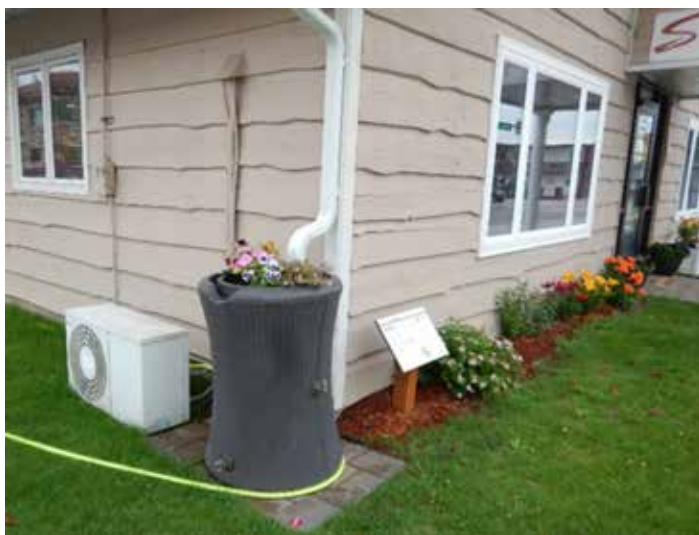
Above: The rain barrel, planters, and pavers at S Salon show how green infrastructure installations and BMPs can help a business look good while reducing their impact on local waterbodies.
