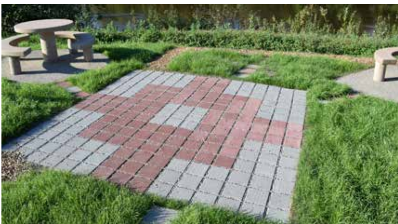
Left: an installation of permeable pavers used to create a patio near the picnic tables, directly adjacent to the Chena River.
