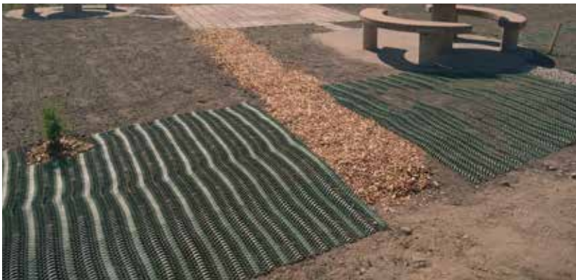
Left: an installation of grass mesh soon after installation and before seed germination. This will help stabilize the lawn near the parking area.
